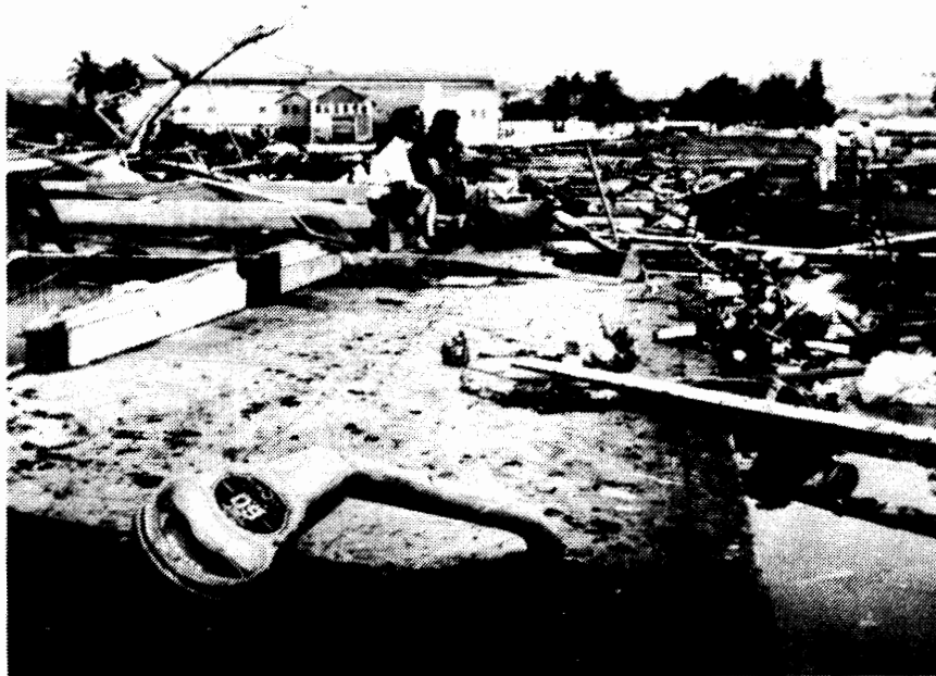
b. Tsunami Damage in Hawaii Following Magnitude-8.5 Chilean Earthquake of May 1960. Aftermath of the Tsunami in the Waiakea Area. Note the Scattered Debris, Gutted Foundation, and the Bent Parking Meters. (Photo Credit: Sunset Newspaper).
