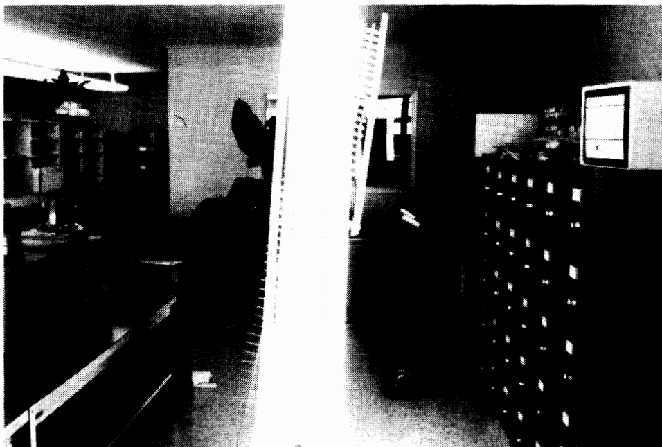
The Life-Threatening Failure of this Fluorescent Light Fixture Is About the Extent of the Disruption in this Office Caused by the Magnitude-6.7 Imperial Valley, California, Earthquake of October 15, 1979. (Photo credit: C. Arnold)
