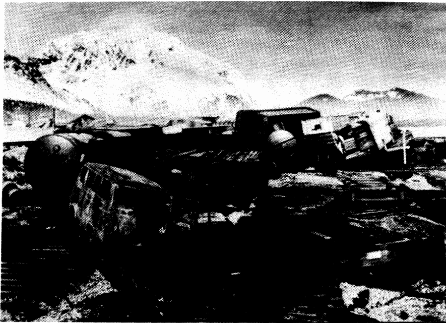
b. Tsunami Damage to the Seward, Alaska, Port Facilities Following the 1964 Alaska Earthquake. (Photo Credit: NOAA/EDS)
