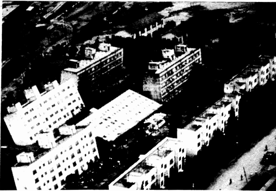
Magnitude-7.5 Niigata, Japan, Earthquake of June 16, 1964. Aerial View of Leaning Apartment Houses Produced by Soil Liquefaction and the Behavior of Liquefiable Soil Foundations. About One-Third of the City Subsided by as Much as Two Meters as a Result of Sand Compaction. (Photo Credit: NOAA/EDS)
