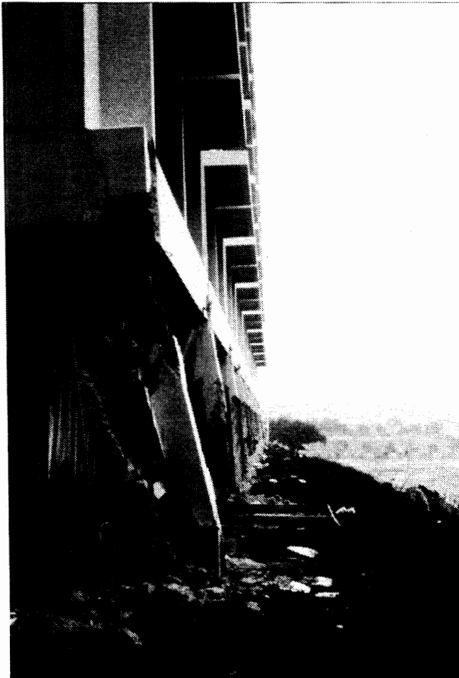
a. Overall View Showing Collapsed End Stairwells, but Generally Good Condition of Upper Portions of Building.
