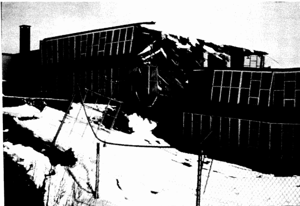
Government Hill School, Anchorage, Destroyed by Landslide During the Magnitude-8.4 Alaska Earthquake of 1964. (Photo Credit: NOAA/EDS)
