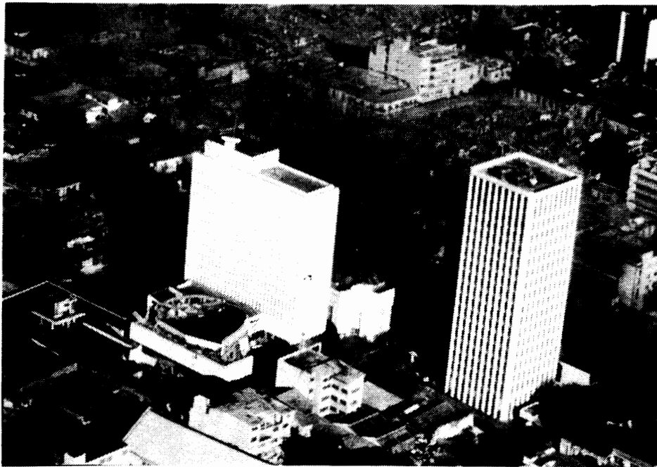
c. View of downtown Managua After the Earthquake Showing the 15-Story Banco Central Building on the Left and the 17-Story Banco de America Building on the Right. The Banco Central, a Reinforced-Concrete, Moment-Resisting-Frame Structure, Sustained Moderate Structural Damage, But Large Interstory Drift Caused Severe Nonstructural Damage. The Banco de America, a Shear-Wall Structure, Sustained Minor Structural Damage, and Only Minimal Nonstructural Damage.
