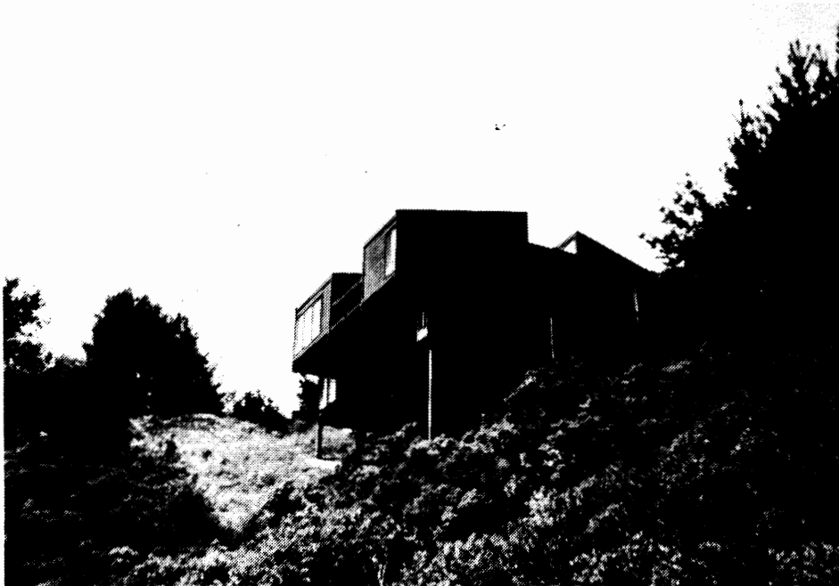
The House on "Stilts", Consisting of Columns Having Little or No Lateral Earthquake Force Resistance Capability, Is Very Vulnerable to Earthquakes.
