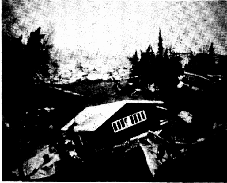
Wood-Frame House in the Turnagain Landslide at Anchorage Following the Magnitude-8.4 Alaska Earthquake of March 27, 1964.
