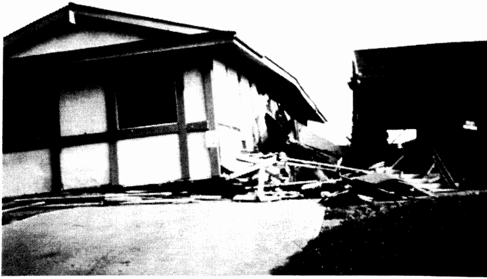
Collapse of a Wood-Frame Split-Level House Following the Magnitude-6.5 San Fernando, California, Earthquake of February 1971. The Cause of This Type of Collapse is the Lack of Shear Resistance of the Garage Door that was Below the Second-Floor Bedrooms and the Lack of Adequate Tying Between the Two-Story and One-Story Portions of the Building.
