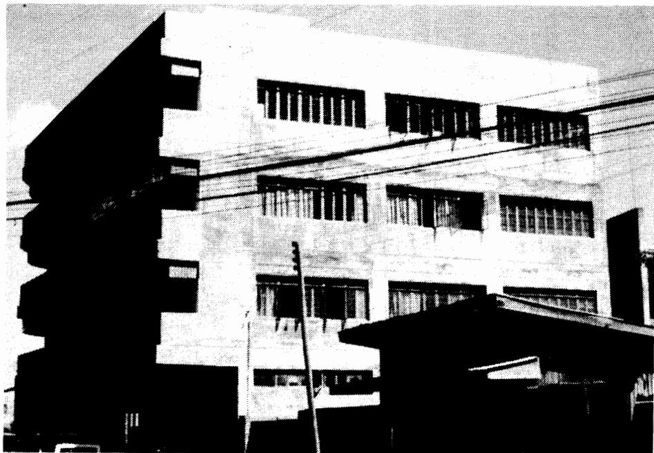
b. The Tison Building, Reportedly the Only Building in Mindanao Designed in Accordance with Seismic Considerations, was Essentially Undamaged.
