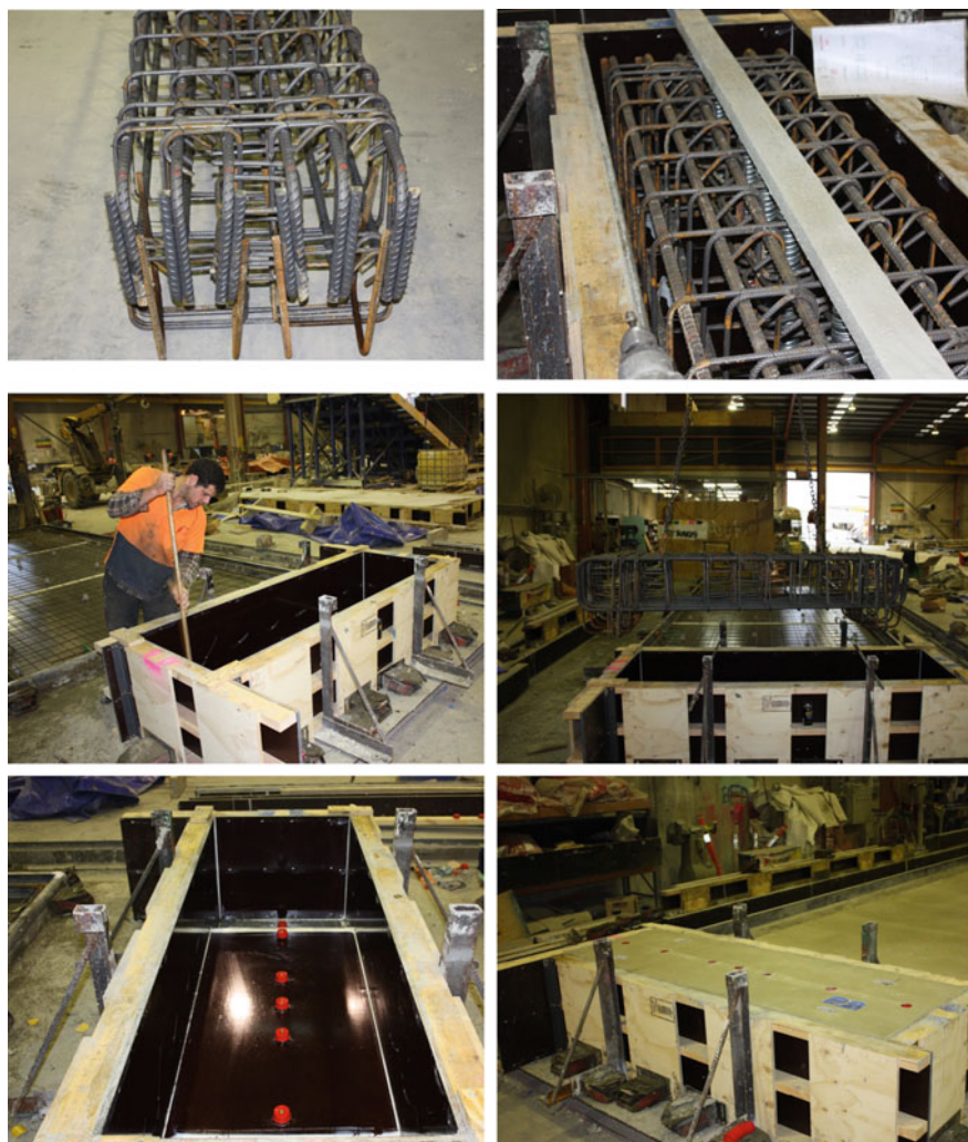
Fig. C.1 Construction of precast concrete footing and loading beam
