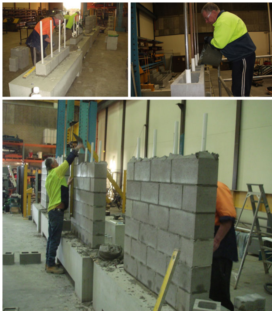
Fig. C.6 Wall construction
