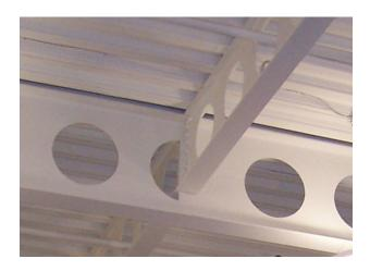
Fig. 2-11. Infill of cellular beam to accommodate a secondary beam.
