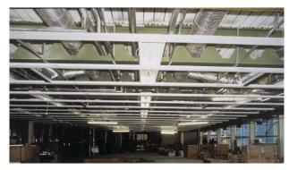
Fig. 2-5. Openings utilized for conduit and HVAC routing.
