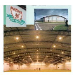
Fig. 2-8. Curved cellular beam roof structure.
