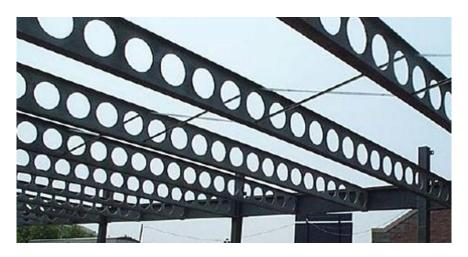
Fig. 2-13. Typical erection bracing for cellular beams (similar bracing used for castellated beams).
