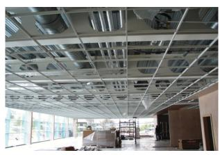
Fig. 2-6. Service integration with ceiling attached to structure.
