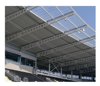
Fig. 2-9. Tapered roof support beams.
