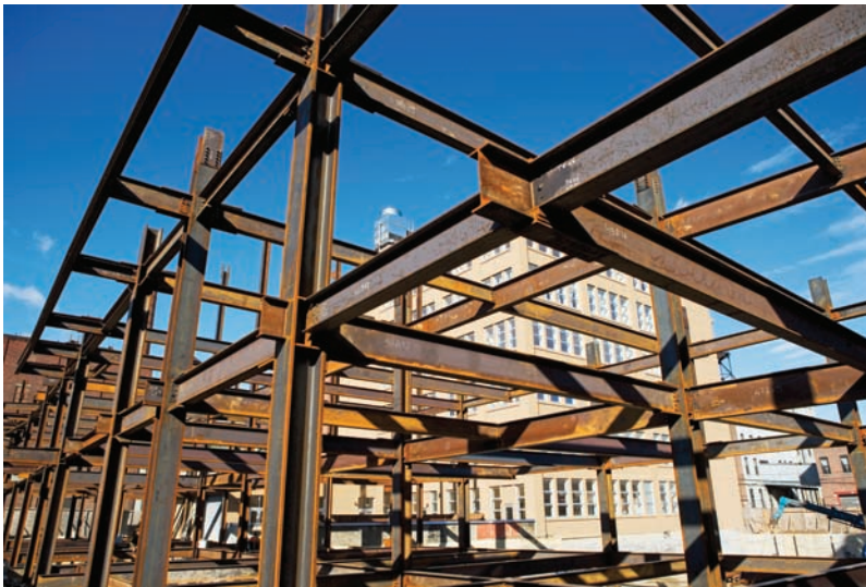
Photo 9.4 The maximum deflection of each beam supporting the floors of a building should be taken into account in the design process.
