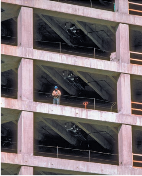
Photo 4.4 Reinforced concrete building frame.
