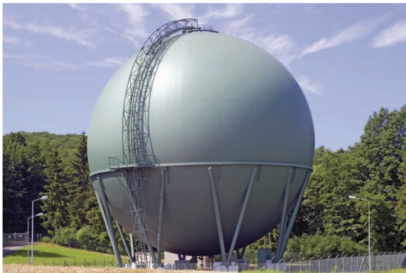
Photo 7.2 Spherical pressure vessel.
