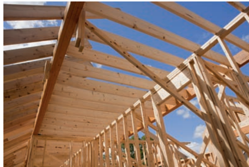
Photo 5.1 Timber beams used in a residential dwelling.
