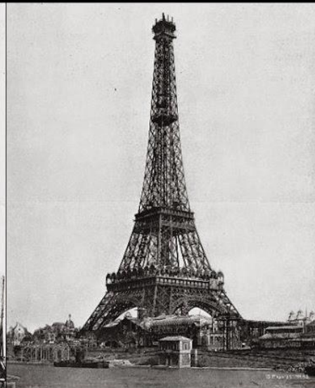
15 MARCH 1889: CONSTRUCTION OF THE CUPOLA
