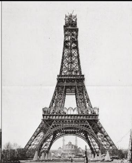
26 DECEMBER 1888: CONSTRUCTION OF UPPER STAGE
