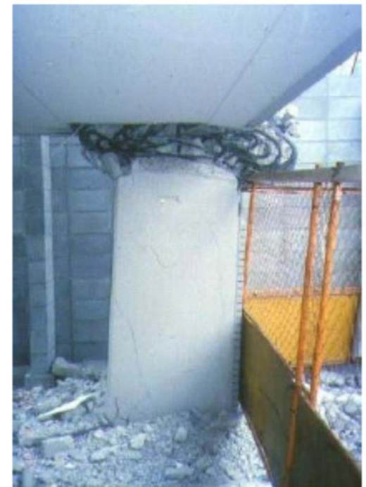
Figure 3 Gravity load collapse from 1995 Kobe Earthquake (AIJ, 1997)
