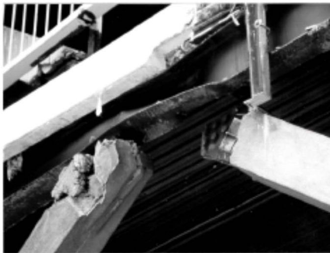
(b) Severe distortion of beam without lateral support at location of chevron braces
