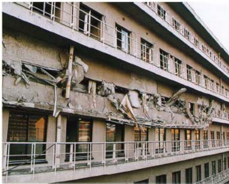
Figure 3 Gravity load collapse from 1995 Kobe Earthquake (AIJ, 1997)
