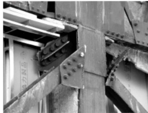
(c) Fracture of welded connection and web tear-out in brace
