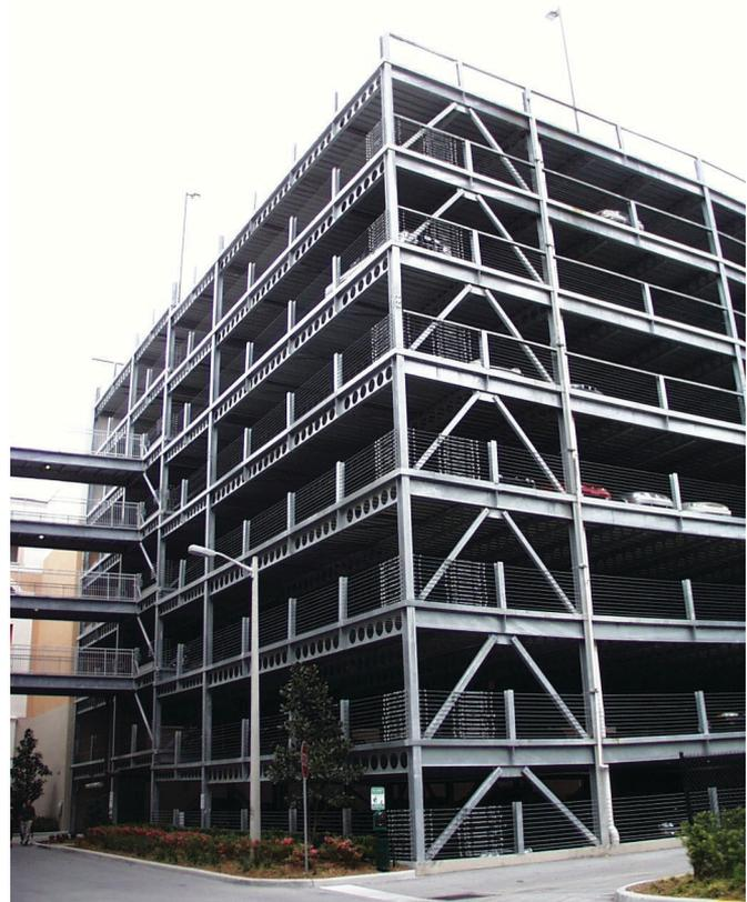
Fig. 2-1. Exterior of parking garage utilizing cellular beams.
