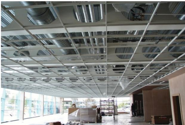
Fig. 2-6. Service integration with ceiling attached to structure.
