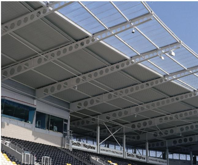
Fig. 2-9. Tapered roof support beams.
