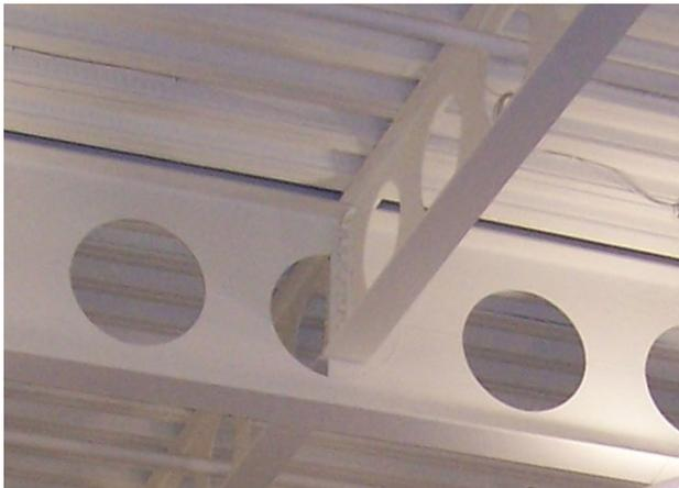
Fig. 2-11. Infill of cellular beam to accommodate a secondary beam.
