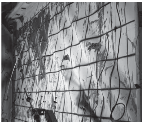
Fig. 2–15. Buckling of infill panel at 1.82 percent drift (Berman and Bruneau, 2003b).
