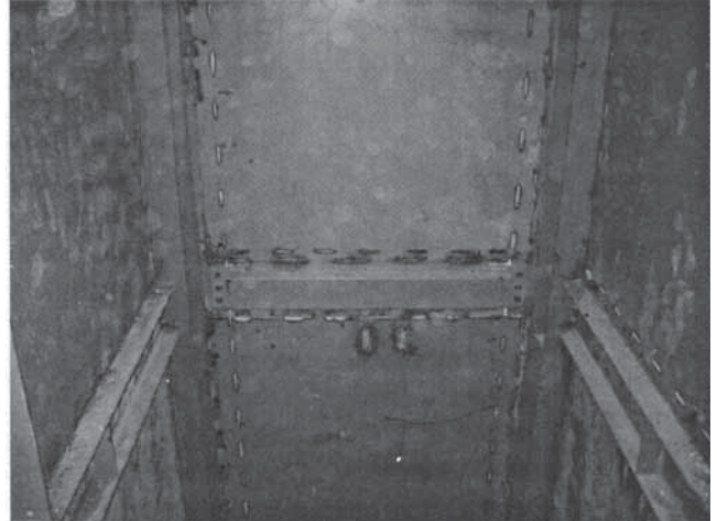
Fig. 1-36. SPW building in Mexico—inside view of walls around elevator core (Martinez-Romero, 2003).
