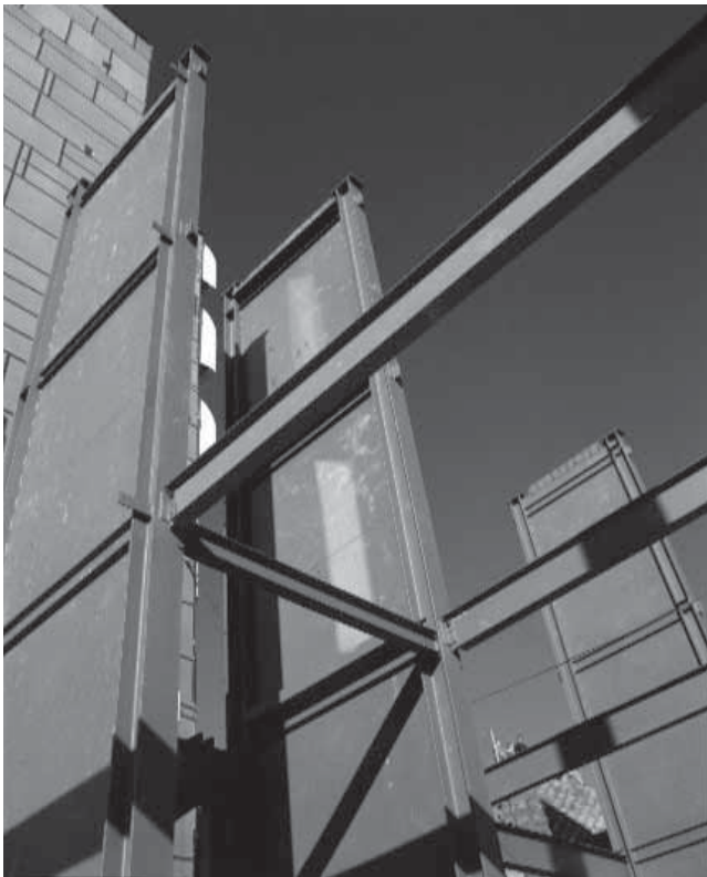
Fig. 1–30. SPW in Canam Manac Group headquarters expansion (courtesy of Richard Vincent, Canam Manac Group, St. George, Quebec, Canada).
