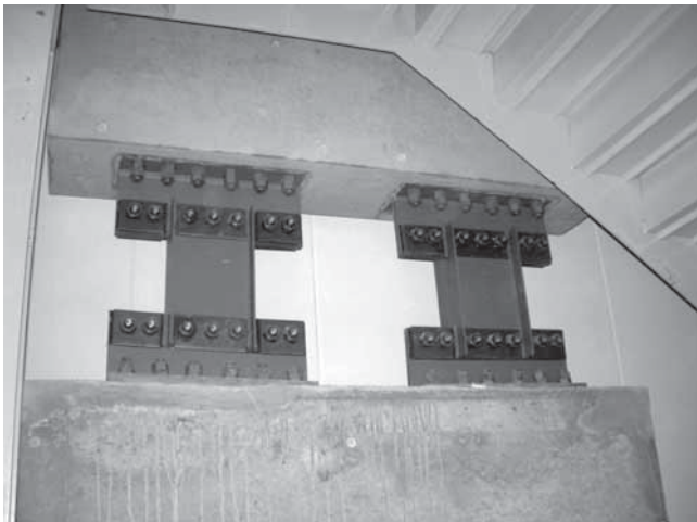
Fig. 1-2. Small shear yielding elements in Japan (courtesy of Shimizu).
