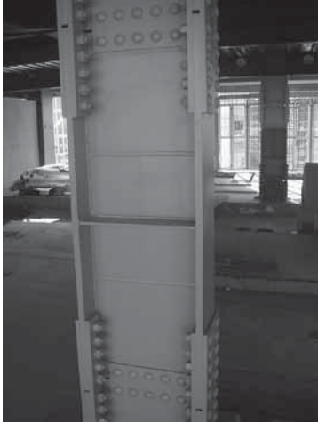
Fig. 1-4. Intermediate column approach used in Japan (courtesy of Takanaka).
