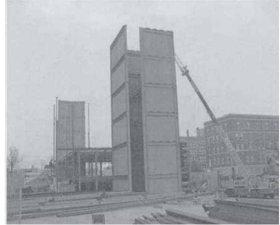
Fig. 1–31. Core wall at middle of ING building (courtesy of Louis Crepeau and Jean-Benoit Ducharme, Groupe Teknika, Montreal, Canada).
