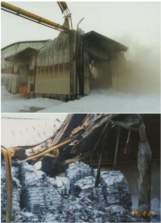
Fig. 11.2 Damage to steel portal frames caused by a fire
