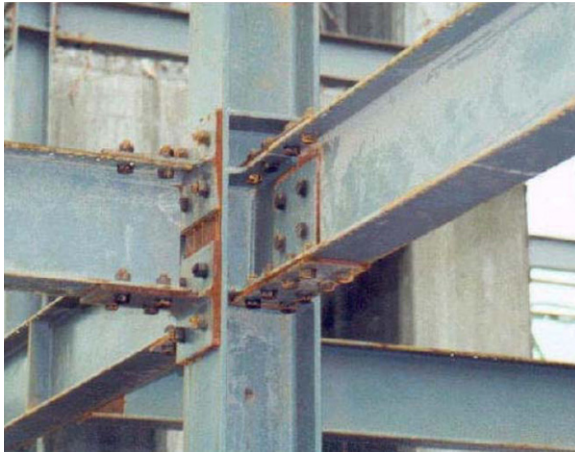
Fig. 8.1 Typical beam-column connection in a framed structure
