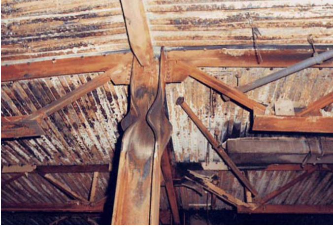
Fig. 1.2 Buckling of the column in a fire
