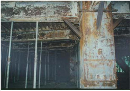
(a) Fracture of the beam-to-column connection
