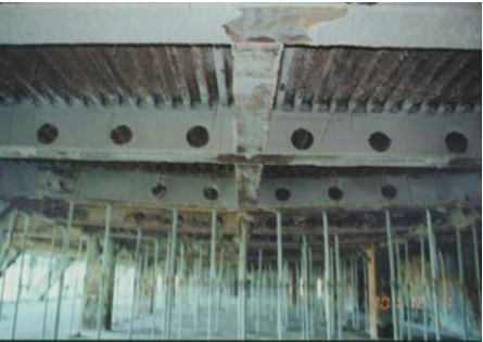
(c) Large deflection in the steel beam
