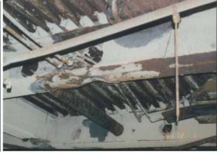
(b) Local buckling of the steel beam
