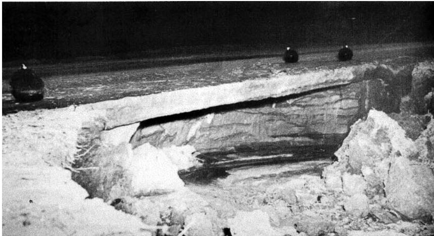
**FIGURE 6.1** Bridging action of soil-cement road surface.
