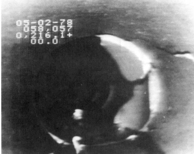
**FIGURE 20.3** Video view of cracked sewer pipe. (Courtesy of Penetryn Systems, Inc., Knoxville, Tennessee.)
