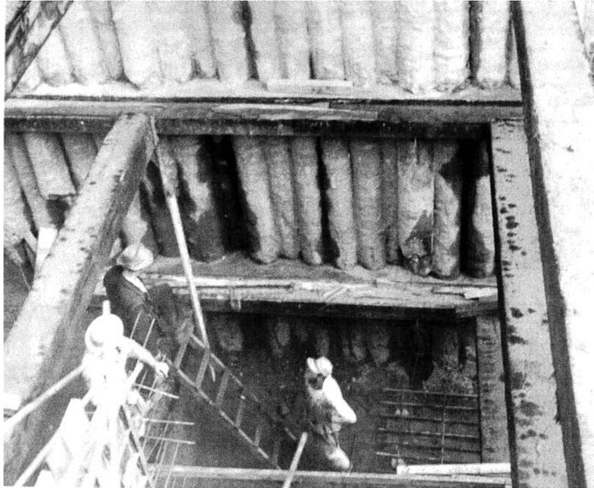
**FIGURE 6.2** Earliest field work with deep soil mixing.
