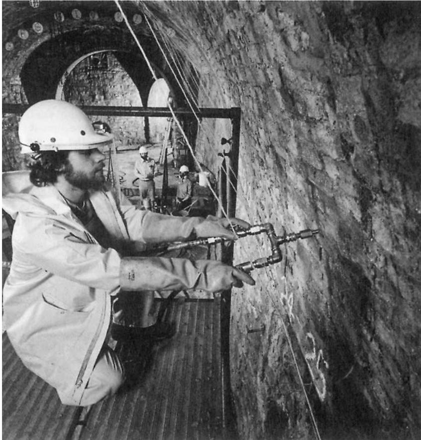
**FIGURE 16.9** Grouting from the inside of a tunnel.
