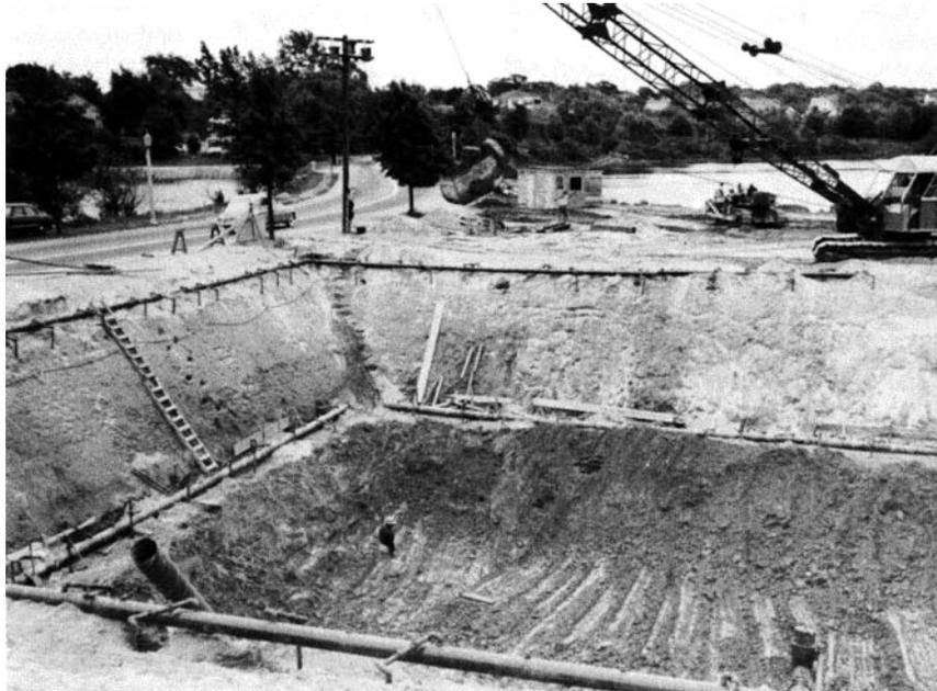
FIGURE 4.8 Wellpoint system in operation.
