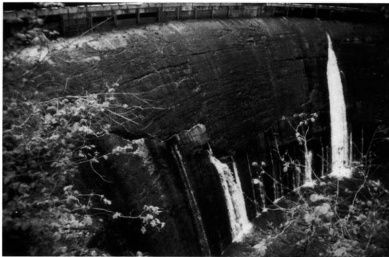
**FIGURE 9.2** Water flowing from large cracks in a concrete dam face. (Courtesy of Engineered Solutions, Inc., Davis, CA.)
