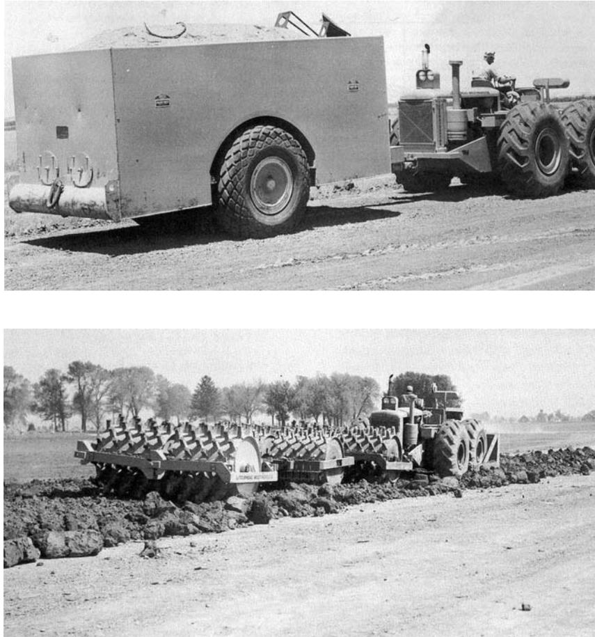
**FIGURE 3.3** Sheepfoot and rubber tired rollers.
