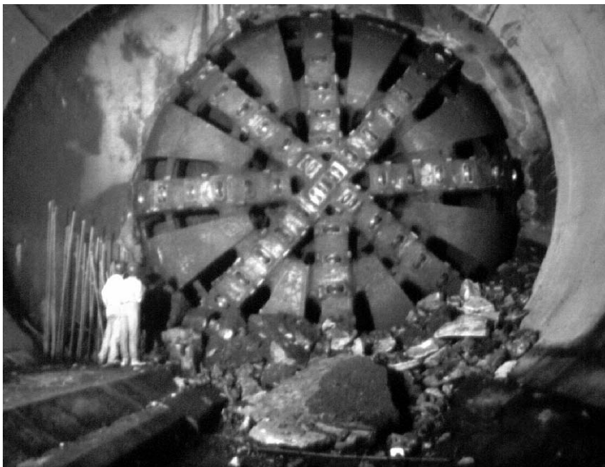
Athens Metro – 9.5m dia. open TBM
