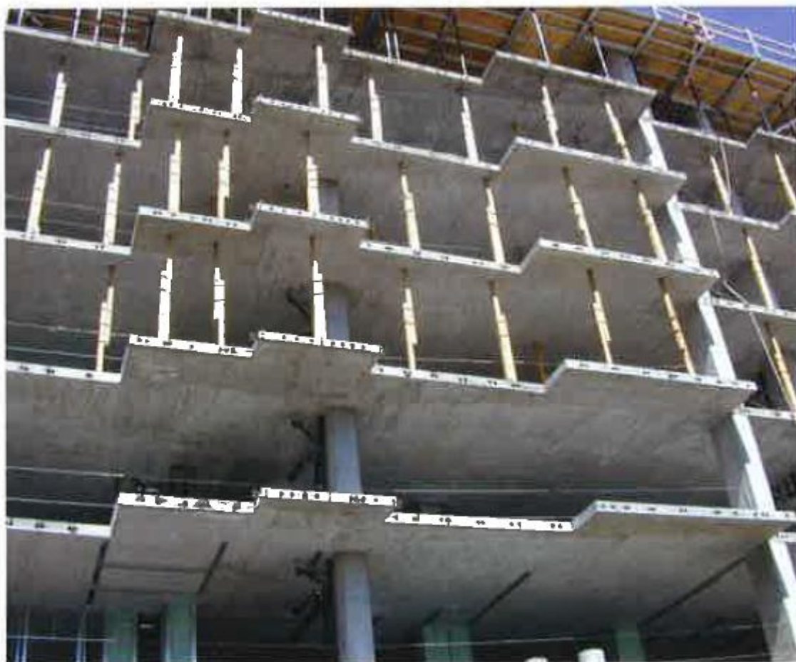
FIGURE 2.2E-1 Beamless Flat Slab Construction Using Post-Tensioning (P134)
