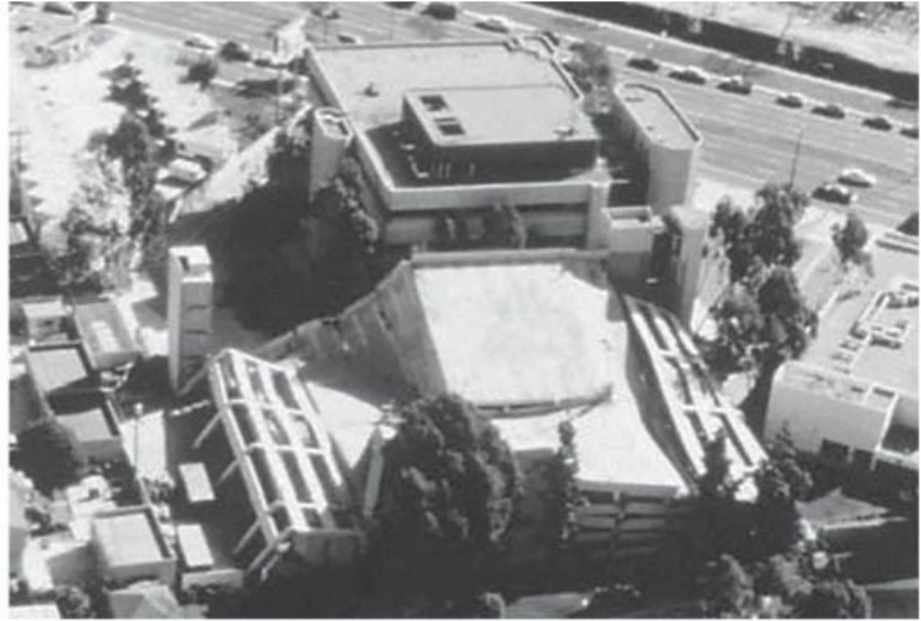
(b) Aerial photograph of collapsed building
