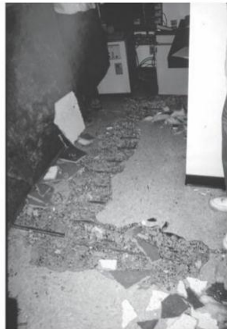
(c) Punching shear failure
