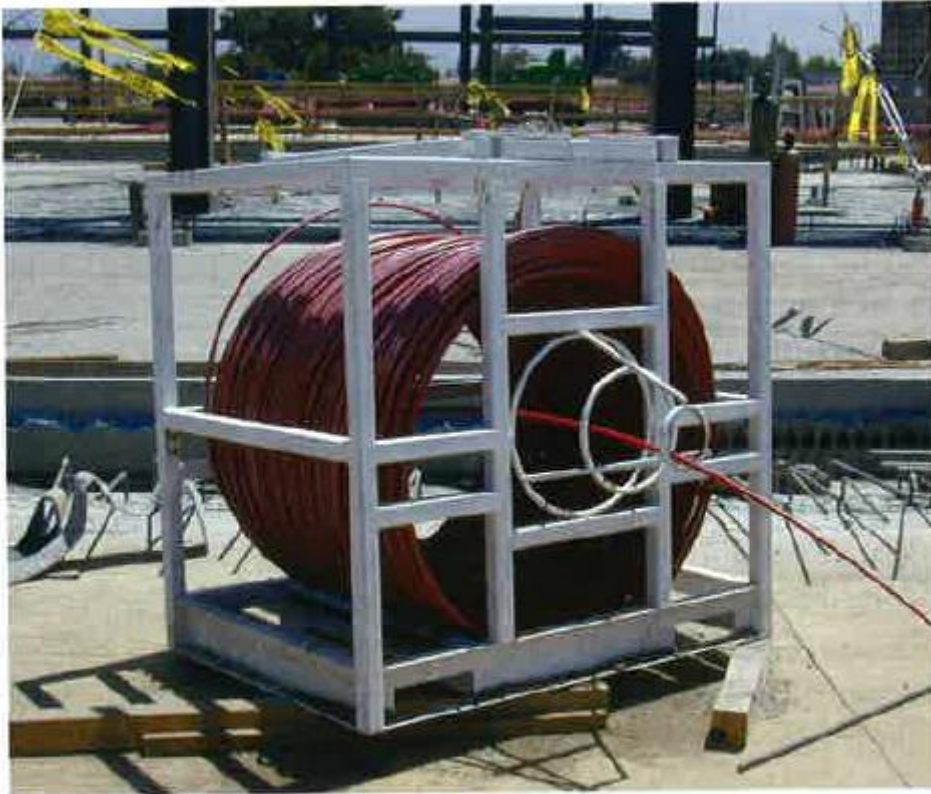
FIGURE 2.5.1A-2 Strand Delivered to Site in Coil (P403)
