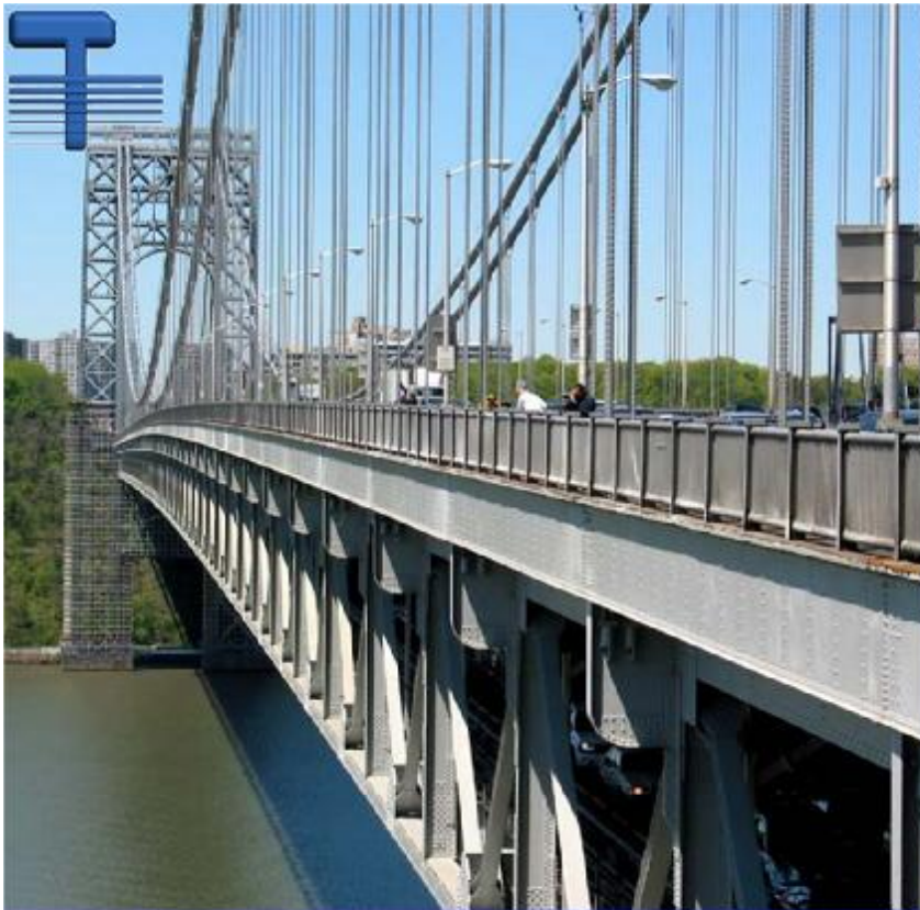
George Washangton Bridge
