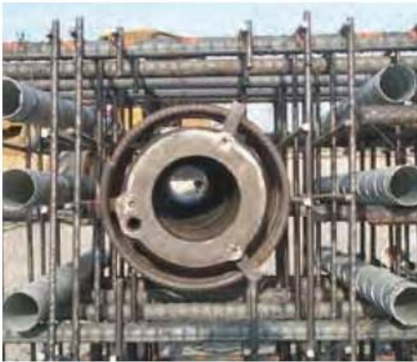
Fig. 8. Reinforcing cage of precast column.
