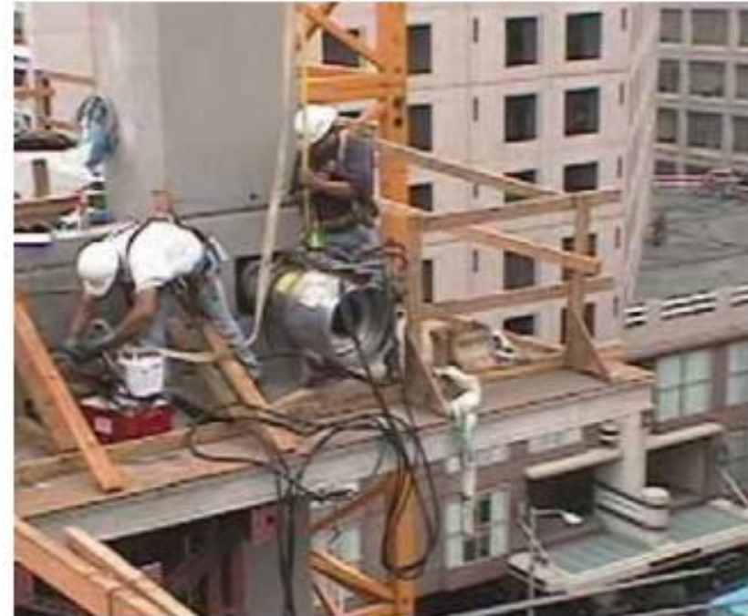
Fig. 11. Jacking operation.
