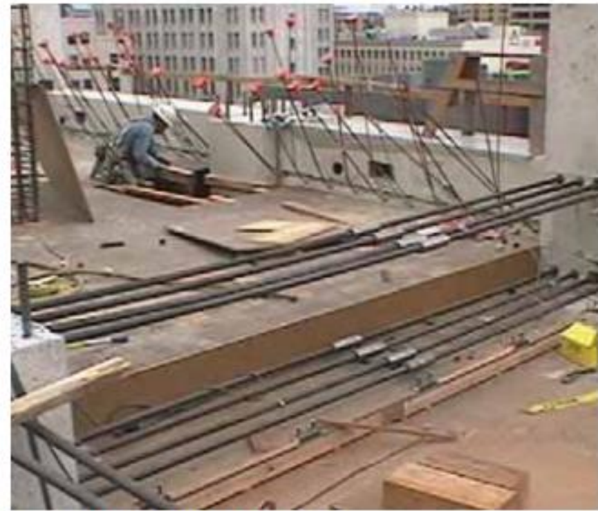
Fig. 9. DDC reinforced frame beam.
