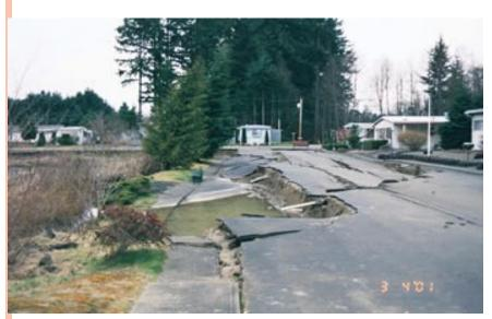
e) Lateral spreading occurs when the soil mass spreads laterally and this spreading comes with tensional cracks in the soil mass.
