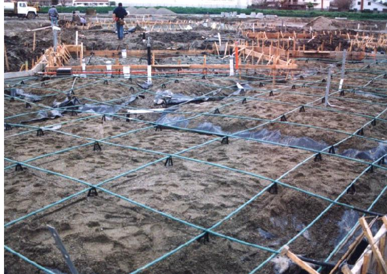
Post-Tensioned ground supported slab (SOG) is the largest application of post-tensioning in USA
