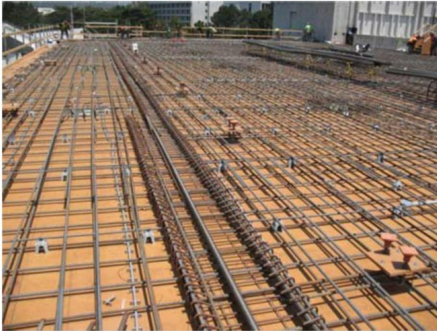
Figure 9-2 – Along collector with confinement reinforcement.
