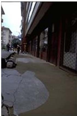
Izmit, Turkey earthquake, Aug. 17, 1999 Magnitude: 7.4
