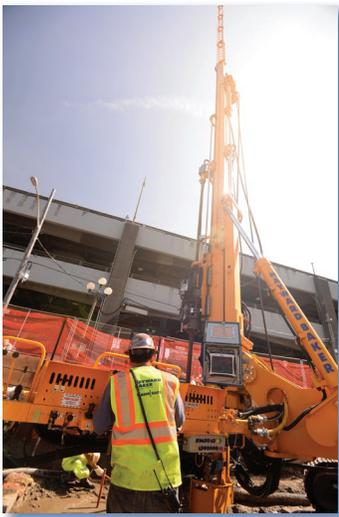
Above: Operator and rig performing jet grouting column installation.
