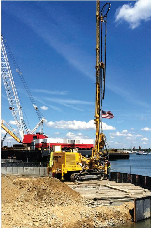
Jet grouting for bulkhead remediation at a marine terminal.
