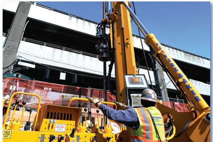
Operator using HBI's proprietary DAQ.
