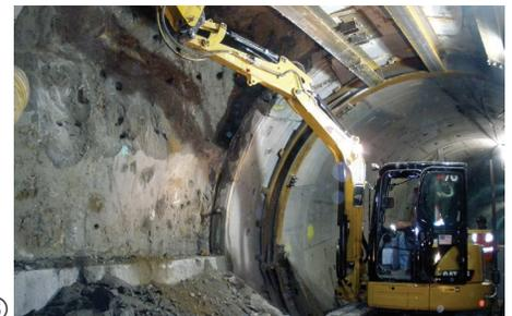
① Jet grout columns used to encapsulate an existing sewer and prevent soil and ground-water from entering the excavation.
