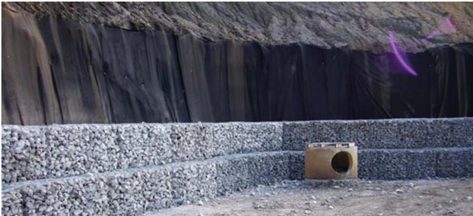
**Fig. 8.20** Geotextile filter behind a Gabion basket wall. (Photo courtesy of Midwest Construction Products, Fort Myers, FL.)
