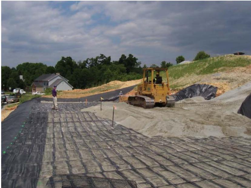
**Fig. 5.38** Example of a reinforced soil slope in construction. (Photo courtesy of Tensar International.)
