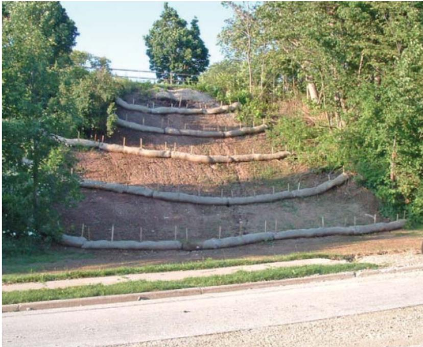
**Fig. 5.28** Surface erosion control using straw tubes.
