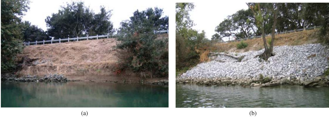
**Fig. 6.11** Rock riprap protection of eroded banks of the Sacramento River (California, USA). (a) River bank erosion (critical condition), (b) river bank after rock riprap repair.
