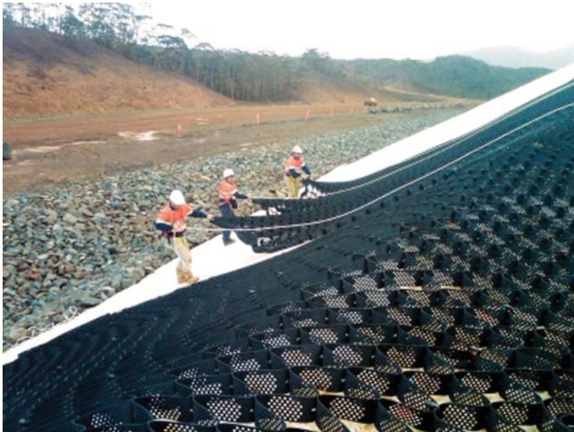
**Fig. 6.12** Geocells are placed on the slope surface and then filled with gravel, as a permanent nondegradable erosion control and slope protection layer. (Photo courtesy of *Geosynthetics* magazine.)
