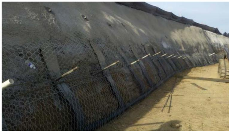
**Fig. 7.4** Soil nail wall used to repair a landslide in Montana, USA. (Photo courtesy of Soil Nail Launcher, Inc.)
