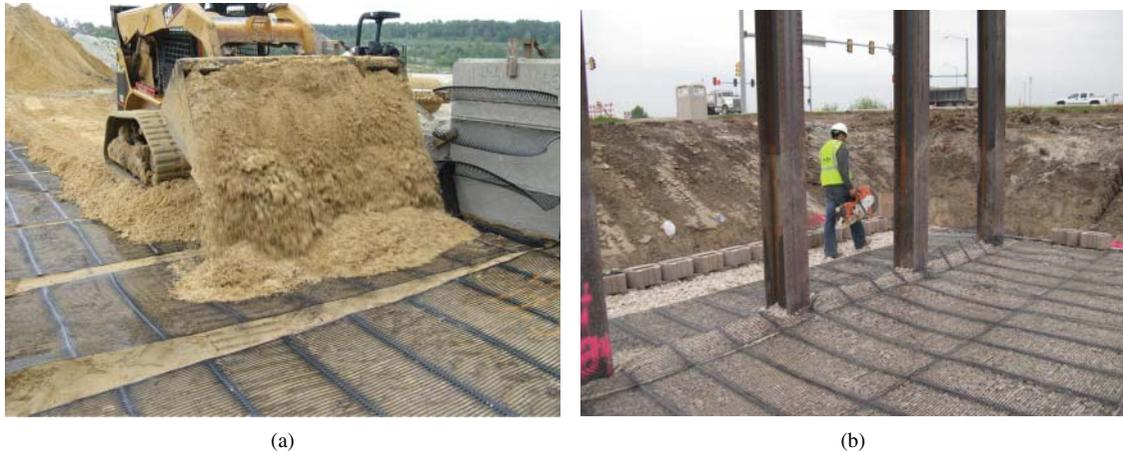
**Fig. 8.3** Examples of construction of MSE wall and abutment. (a) MSE wall, (b) MSE bridge abutment. (Photo courtesy of Tensar International.)
