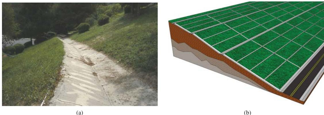
**Fig. 5.27** Slope surface drainage. (a) Interceptor trench drain, (b) interconnected surface drains.
