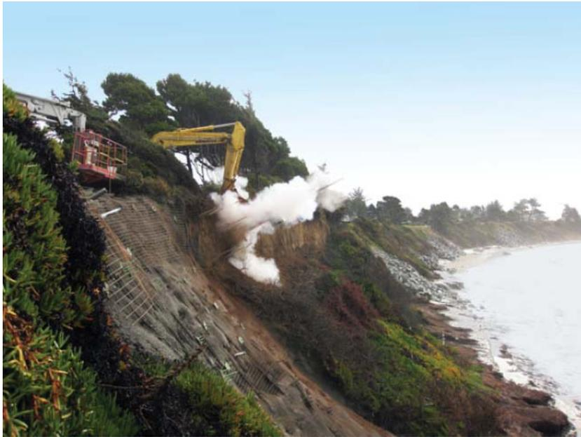
**Fig. 7.38** Soil nails are used to stabilize the bluff at Pebble Beach Drive, Crescent City, California. (photo courtesy of Soil Nail Launcher, Inc.)
