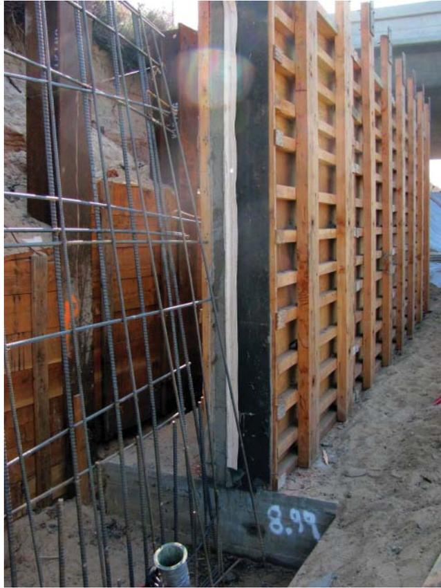
**Fig. 7.19** Conventional retaining wall construction process (Highway 41, Fresno, California, USA, 2010).
