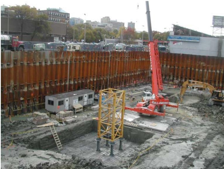
**Fig. 7.2** Sheet pile wall for vertical cut. (Photo courtesy of Earthwork Engineering, Inc. Hollis, New Hampshire.)
