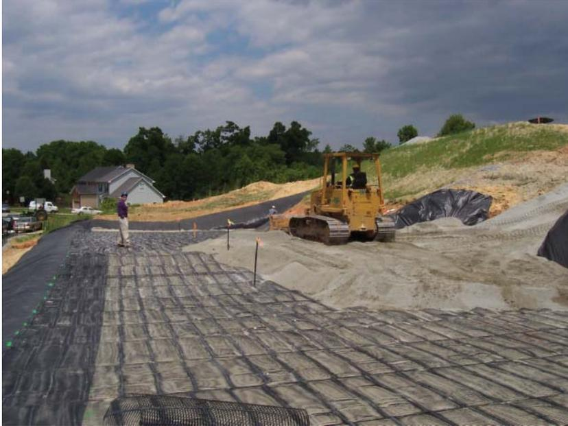
**Fig. 8.11** Example of a reinforced soil slope in construction. (Photo courtesy of Tensar International.)
