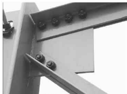
Figure 7-17. Misc. Connection: Truss Column C2 / Truss B7
