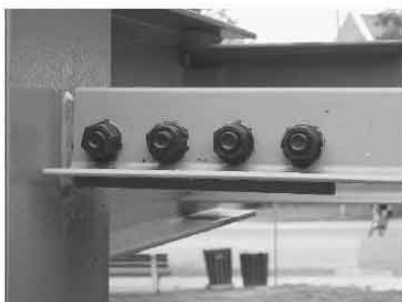
Figure 7-18. Misc. Connection: Truss Column C2 / Truss B7
