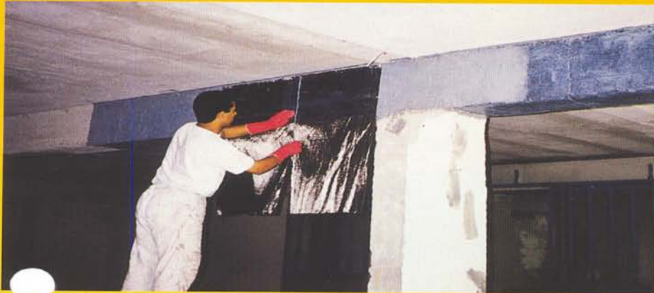
Shear strengthening in a building.
