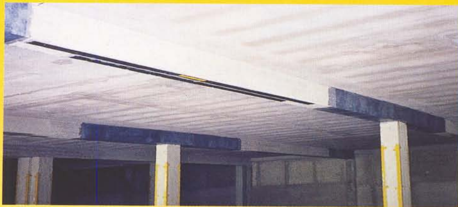
Shear strengthening overview.
