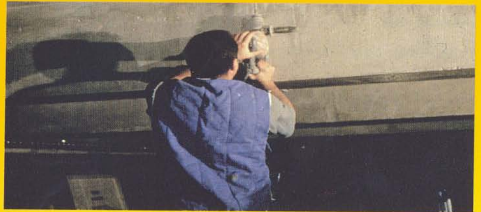
Surface preparation and sealing cracks with Sikadur ® injection.
