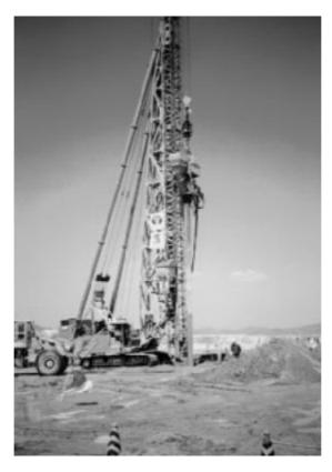
*Figure 11.36* Sand drain installation in progress (*Courtesy of E.C. Shin, University of Inchon, South Korea*)
