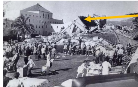
Partial Collapse of Hospital
