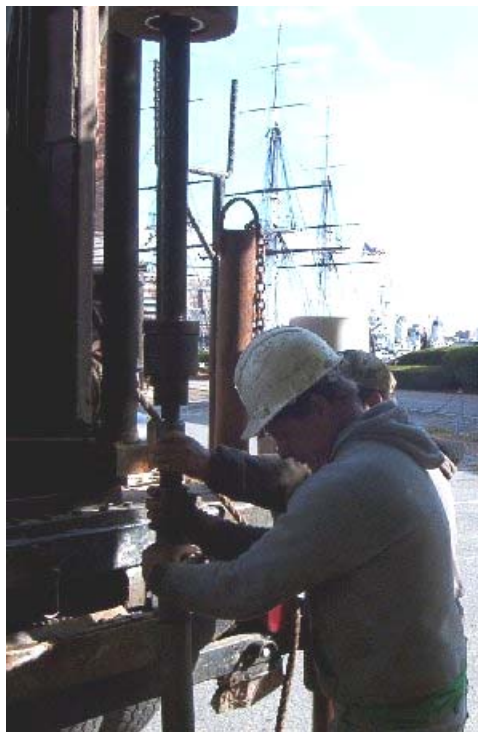
Photograph 2.2 – Standard Penetration Test
