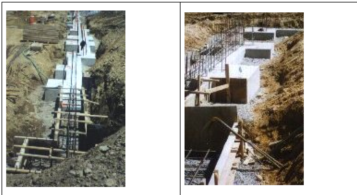
Photograph 4.1 – Shallow Spread Footings
